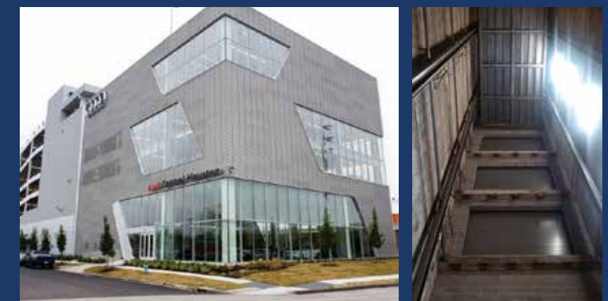
Auto Dealership High Rise Lift – F Series Mechanical VRC High-capacity lift moves luxury automobiles to storage and service levels. 8,000 lbs. lifting capacity; 73' lift travel; 6 levels of service.
